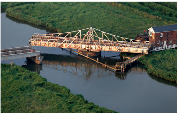
Somerleyton swing bridge – image courtesy of Mike Page – www.mike-page.co.uk
