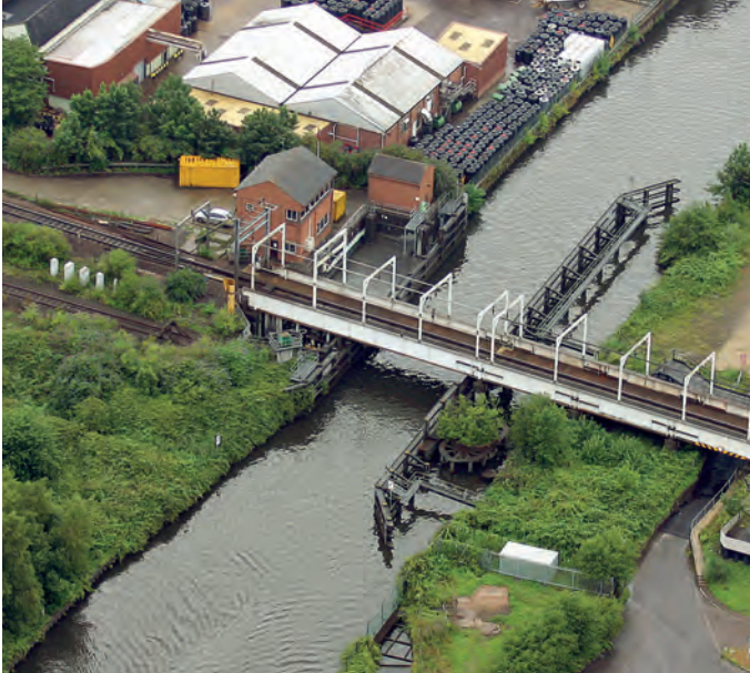
Trowse swing bridge – image courtesy of Mike Page – www.mike-page.co.uk
