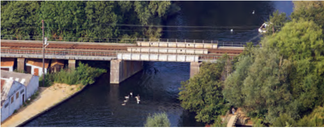
Wroxham rail bridge – image courtesy of Mike Page – www.mike-page.co.uk
